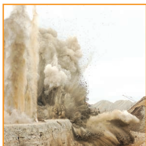
The Boretrak system enables faster yet safer rock face blasting.
