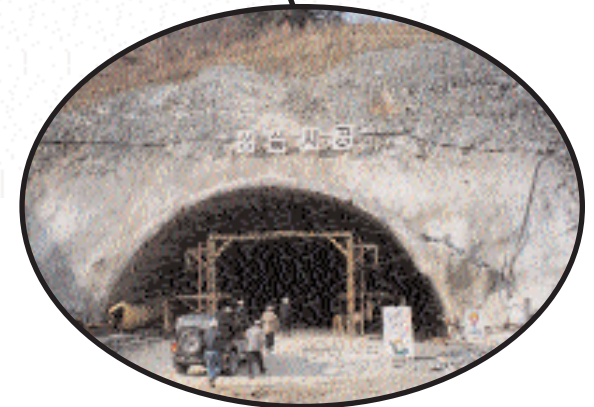
The entrance to one of the two parallel tunnels
