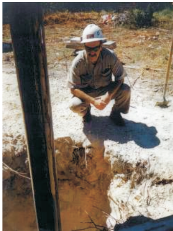
Installation of a utility pole
